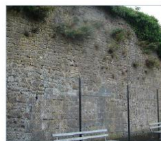
Wall at GAA pitch
