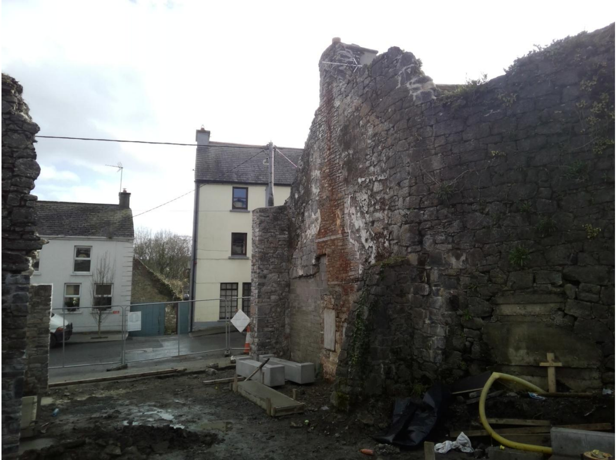
Pic 8: Section of wall at entrance to new park from Burke St. The gable wall and upper portion of the town wall have been partly conserved. There is a blockwork infill panel at the base of this wall, which will be finished with a lime harling as part of the proposed works.
